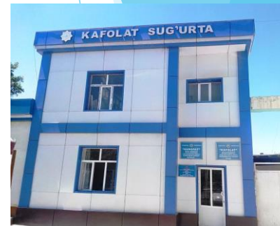
Termez city branch office
