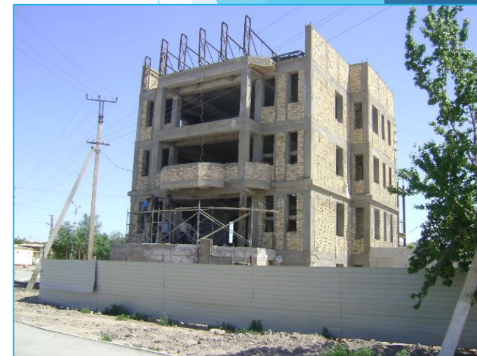
Construction of branch office building in Urgench city
