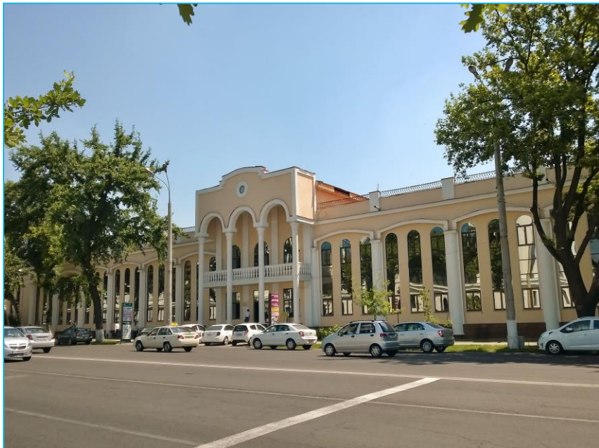
Reconstruction of the Head Office (Board) building in Tashkent city.
