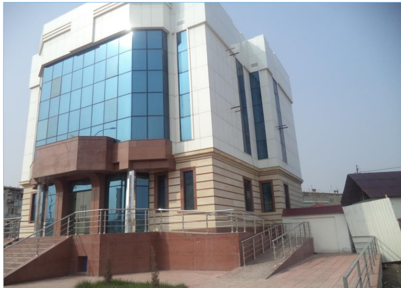
Completion of construction of branch office building in Fergana city
