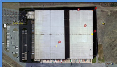
Thermal Anomalies are Pinpointed
