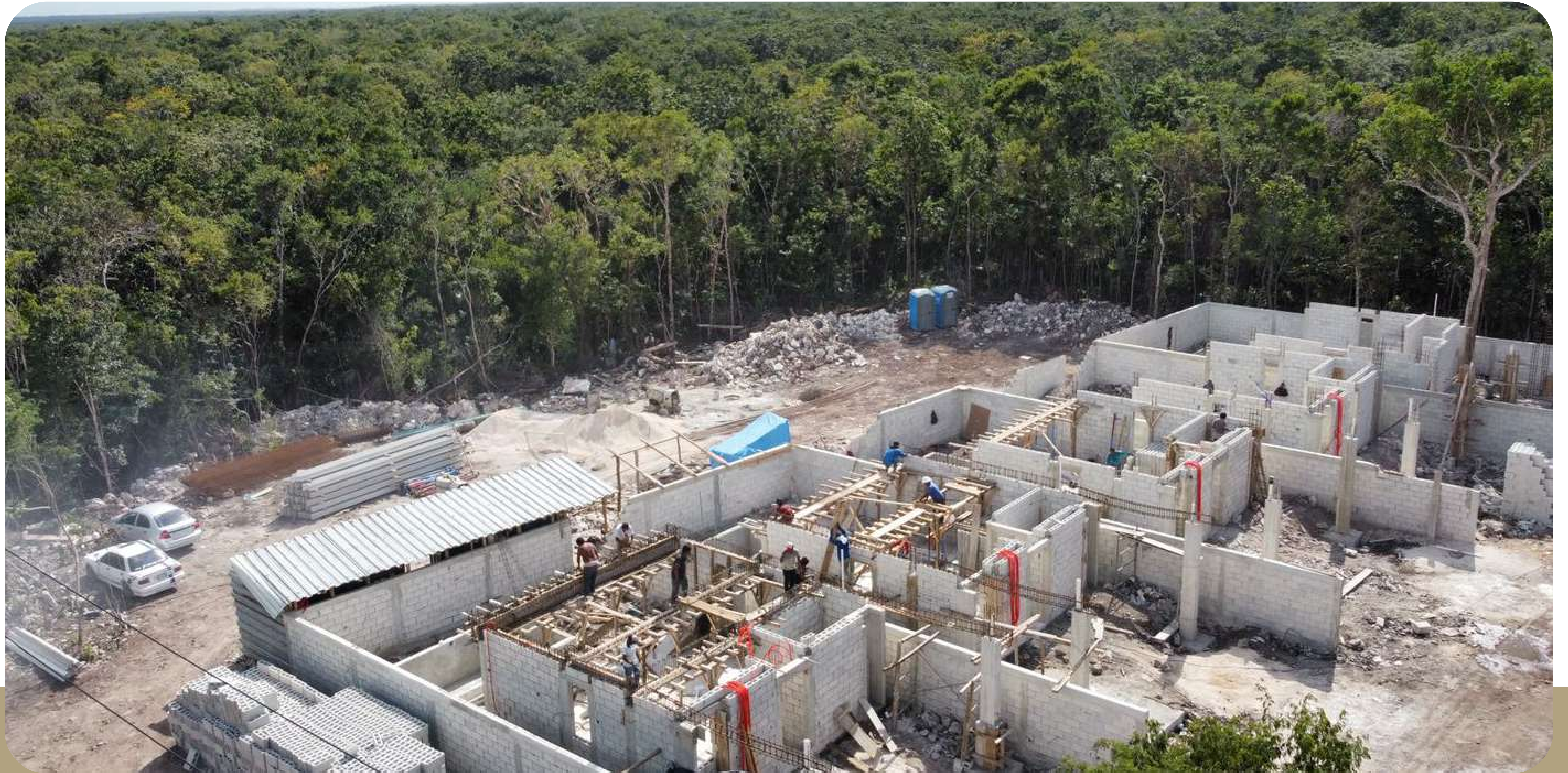
Ground Floor Construction
