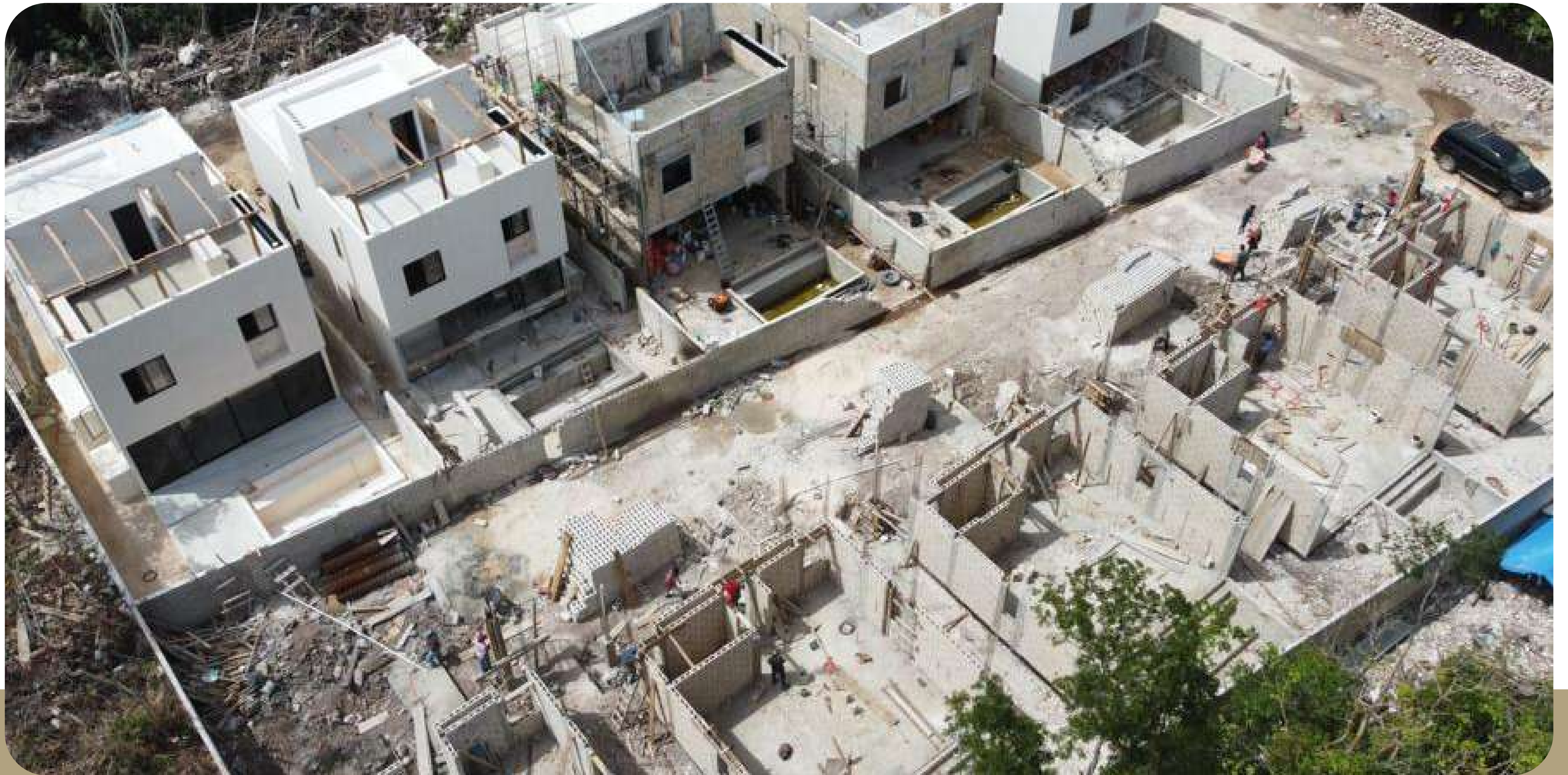
First Floor Construction
