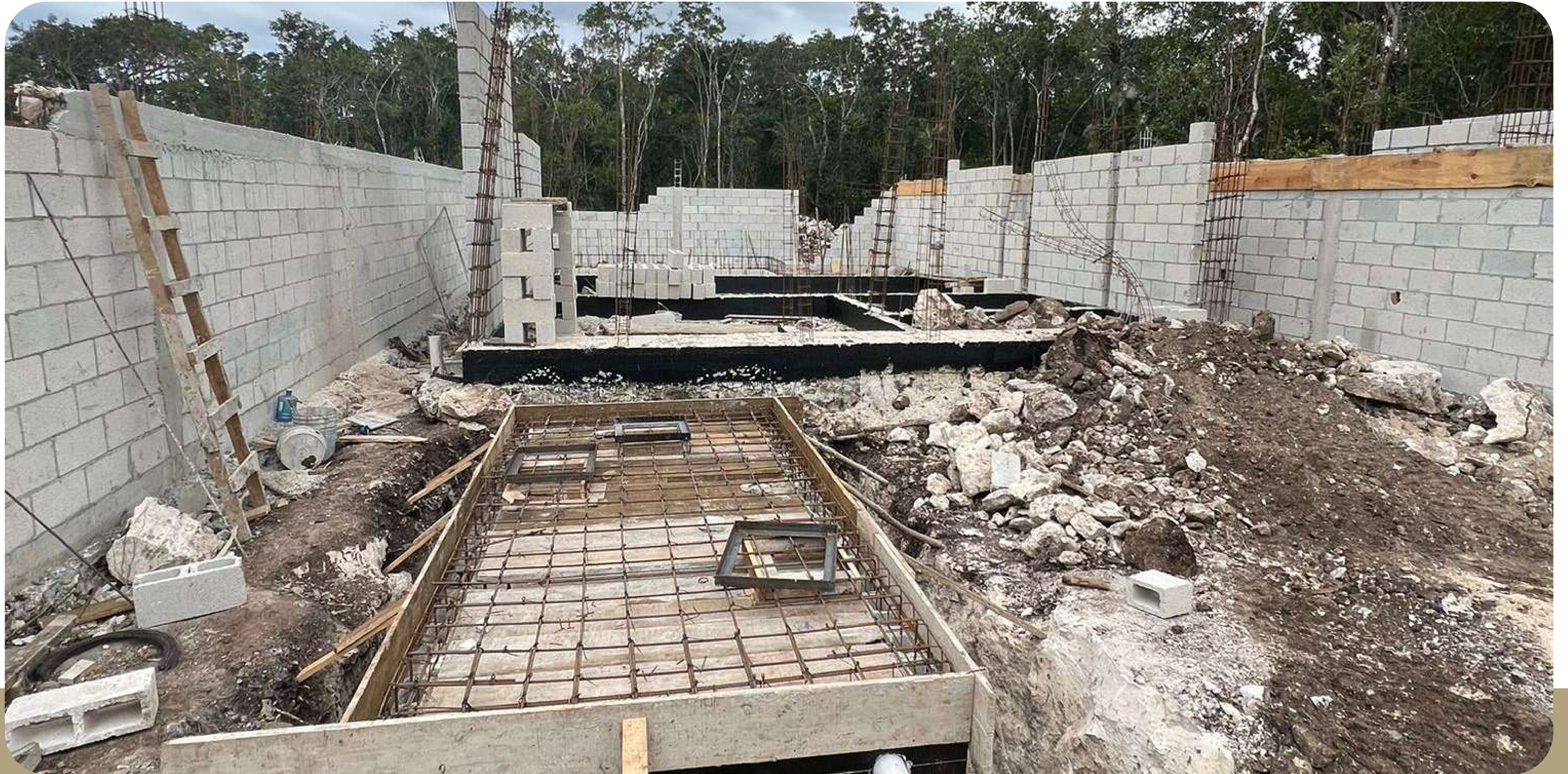
Ground Floor Construction
