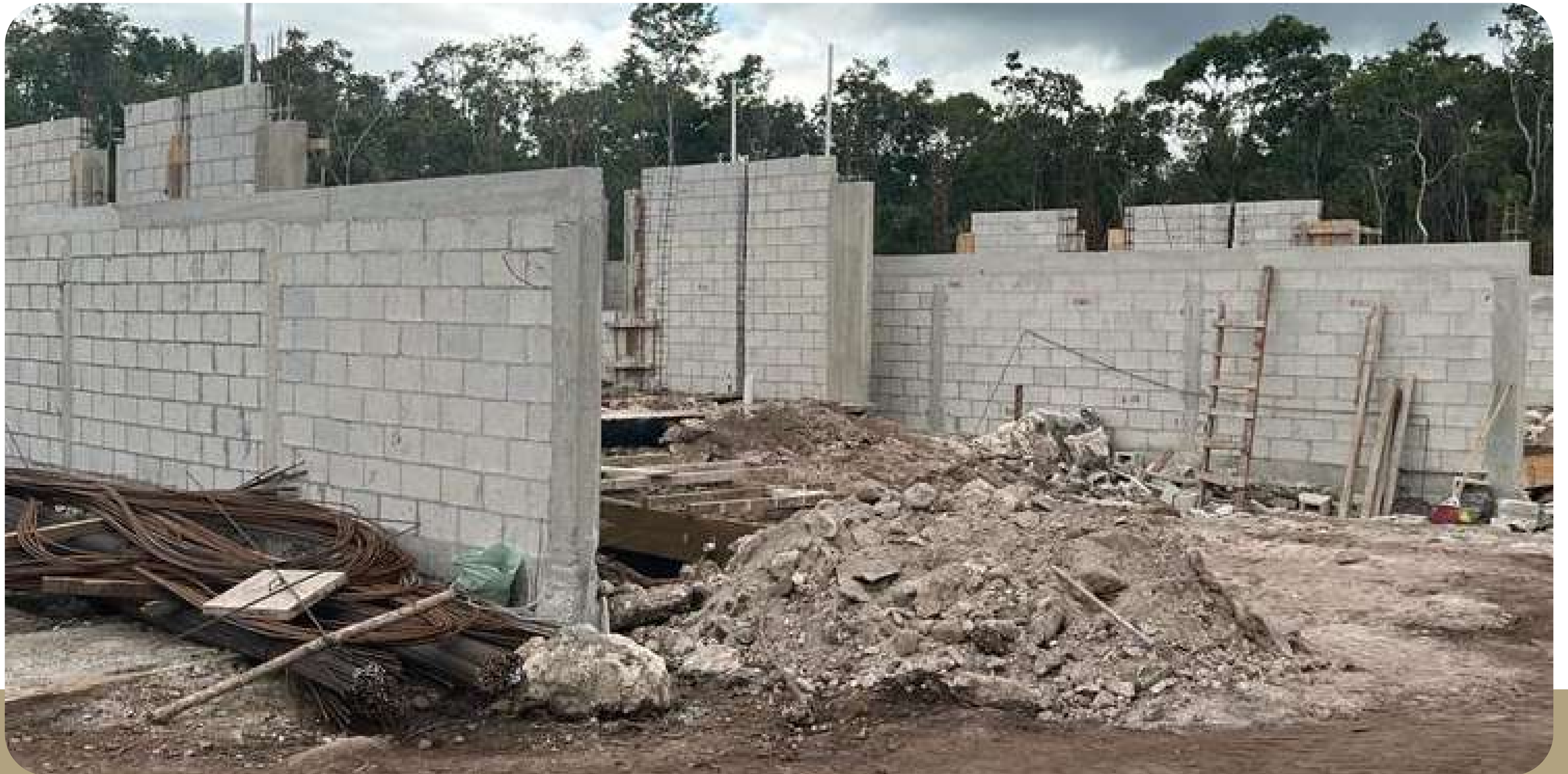
Ground Floor Construction
