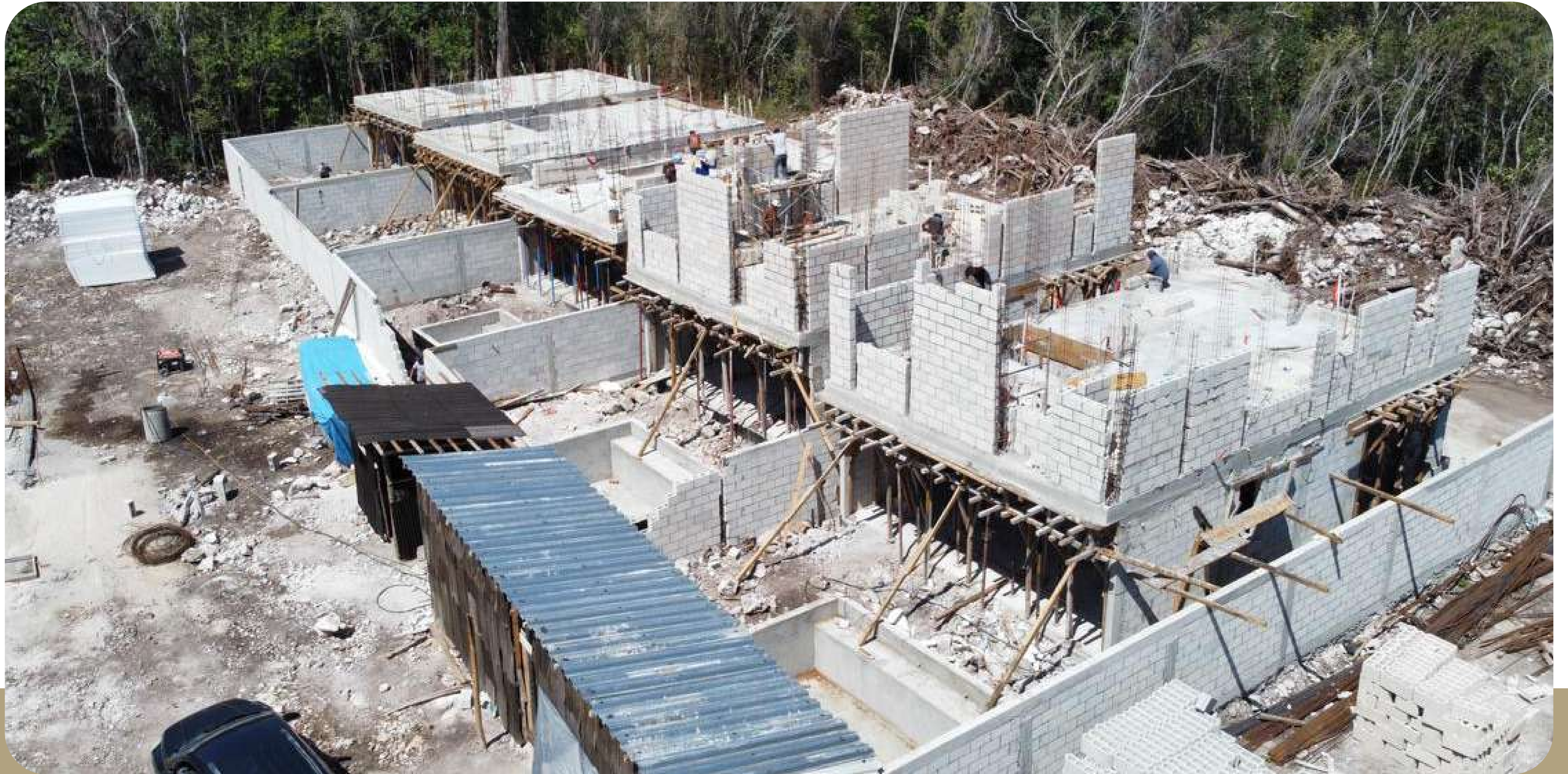
First Floor Construction
