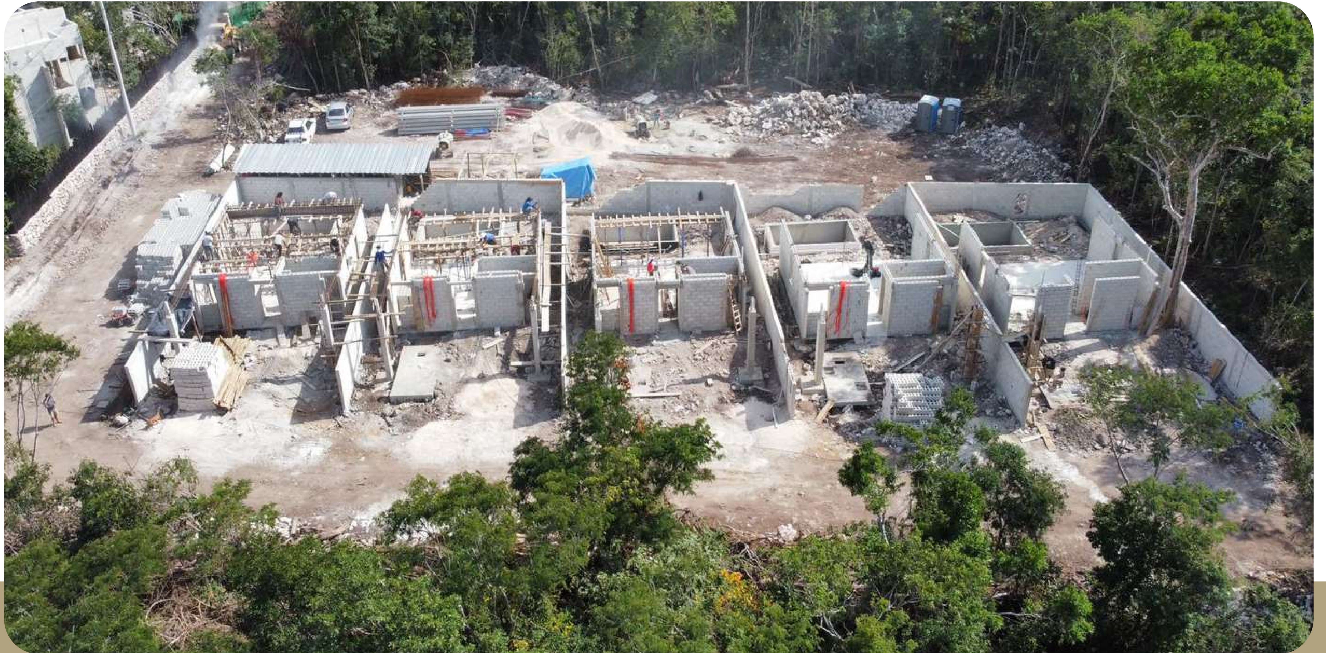
Ground Floor Construction
