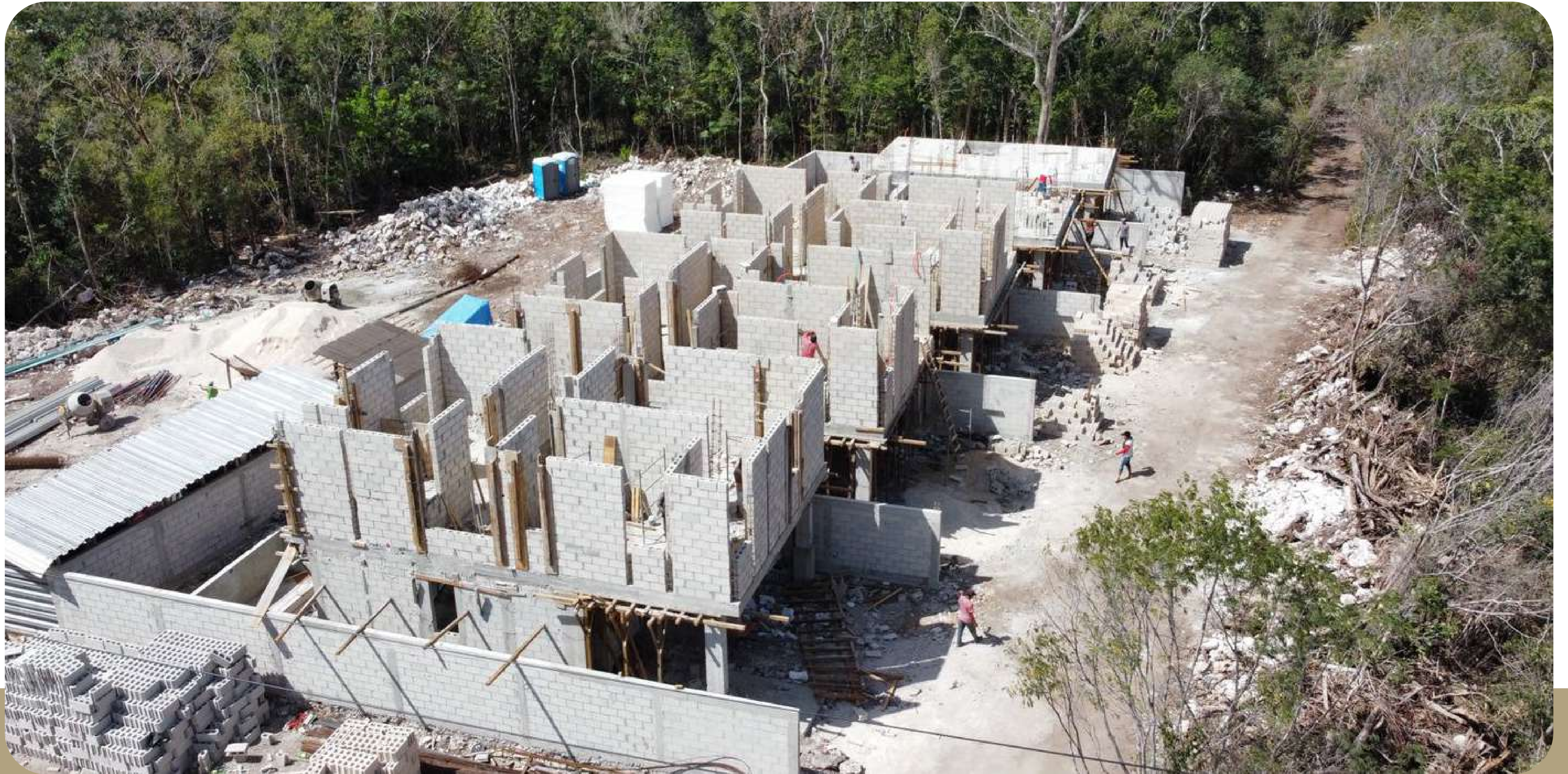
First Floor Construction
