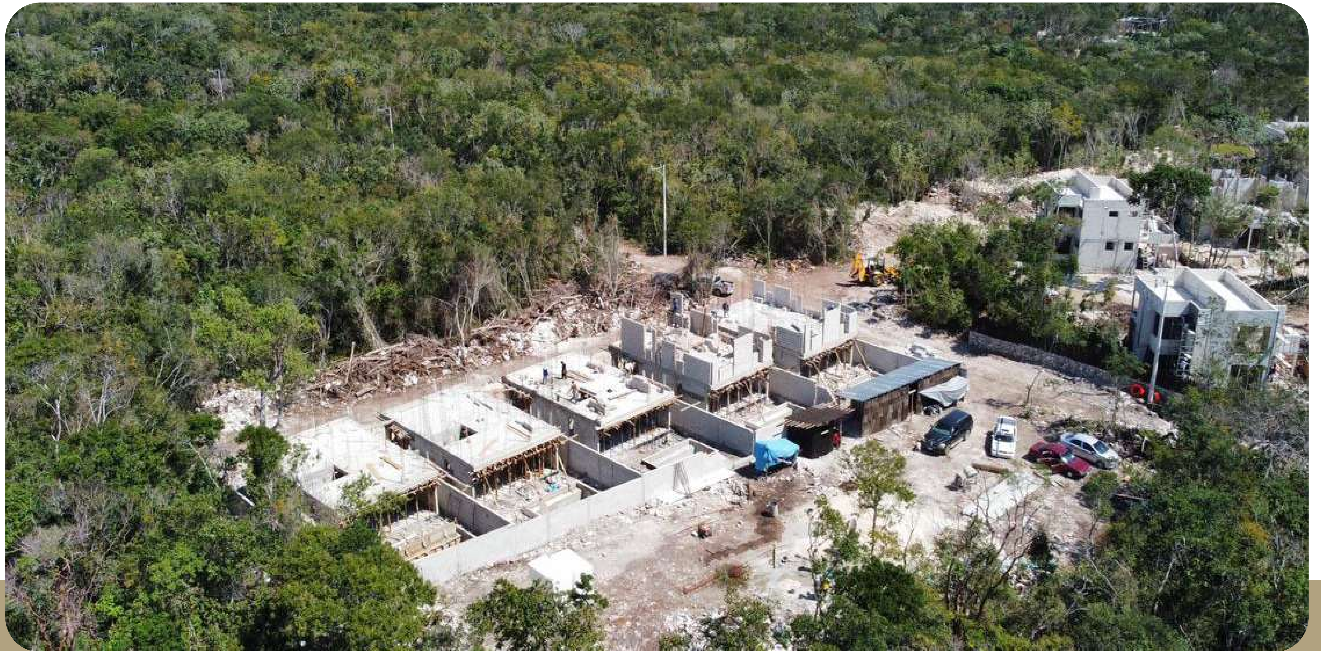
First Floor Construction
