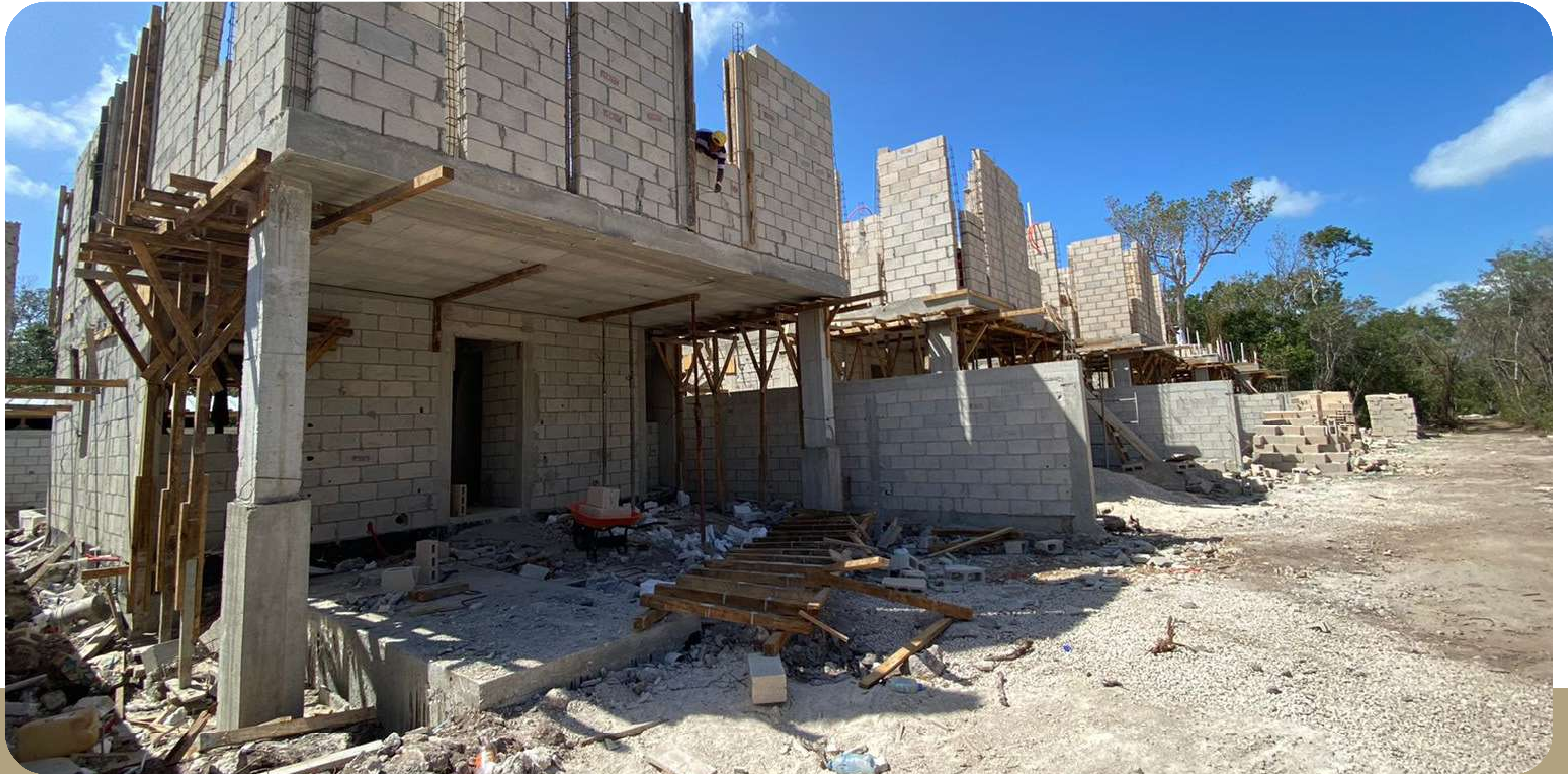
First Floor Construction
