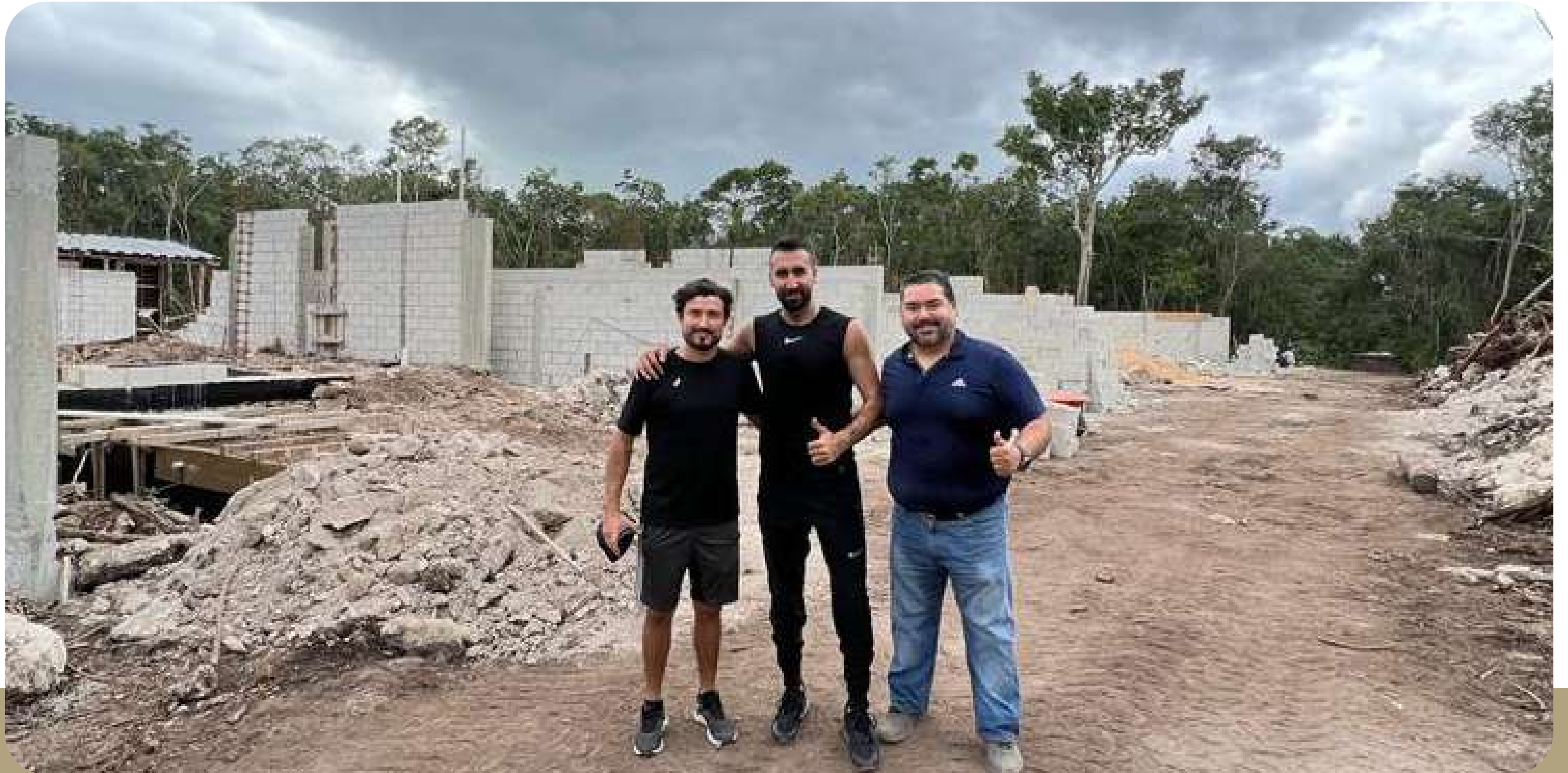
Ground Floor Construction
