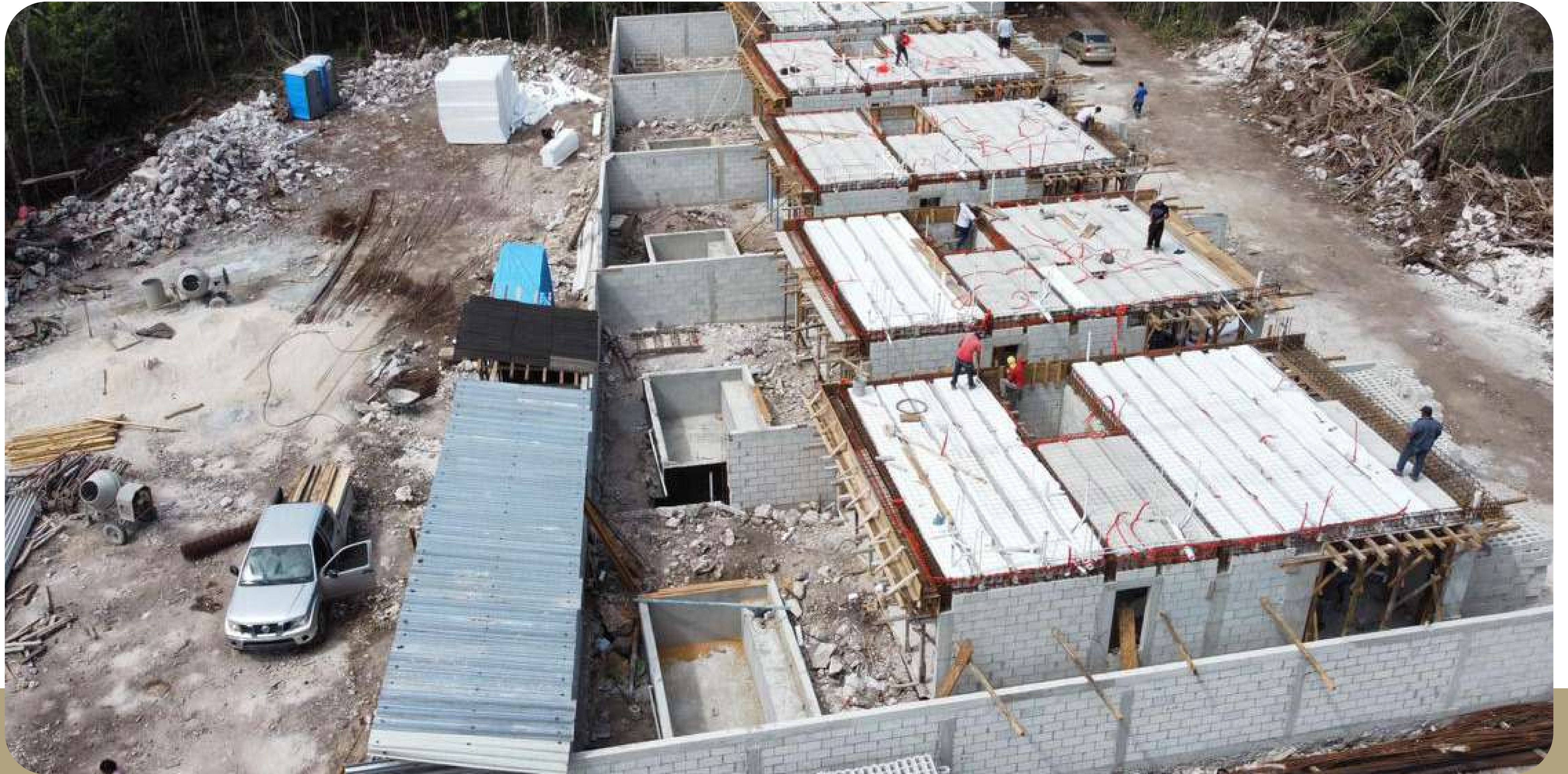
First Floor Construction
