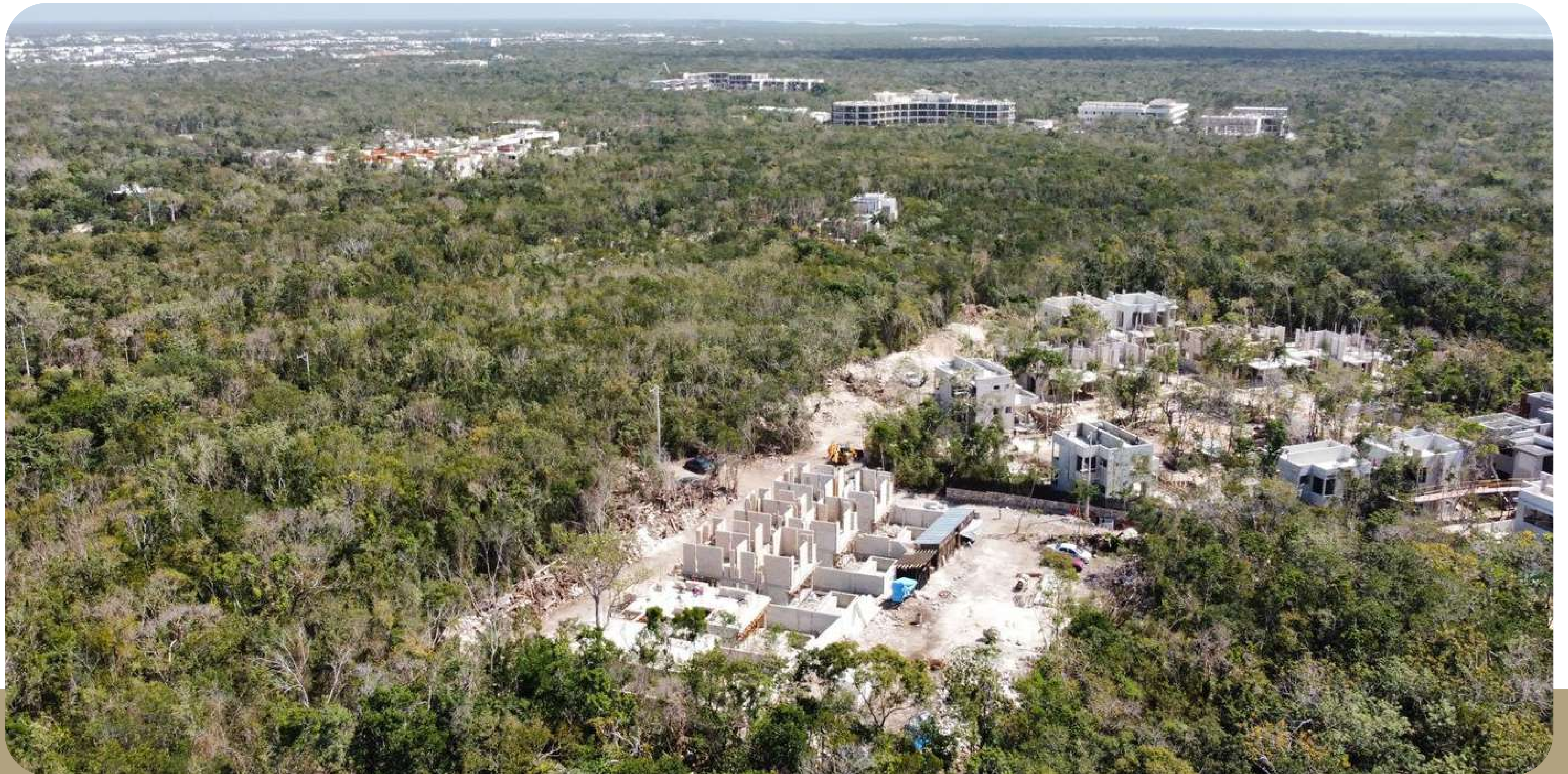
First Floor Construction
