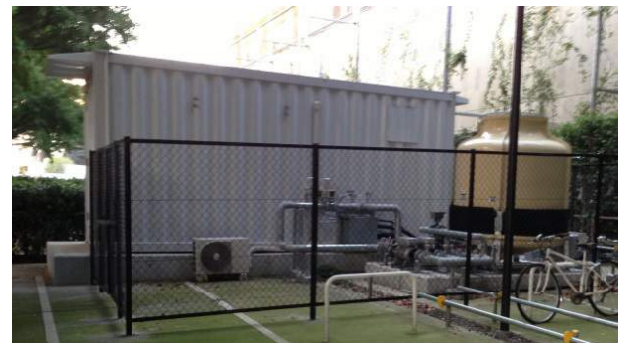
Fig. 3. Exterior view of TSUBAME-KFC: evaporative cooling tower right next to the 20-foot container for complete lights-out operation and low waterpump power
