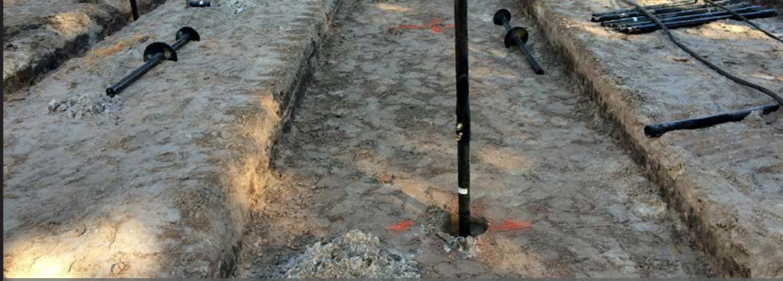
Installation of helical piles to support home's foundation
