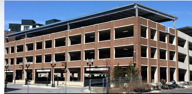
Parking Garage Canopy
