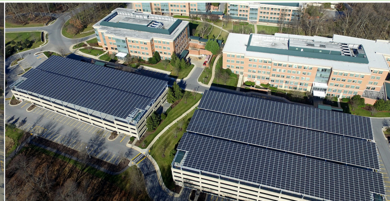
Parking Solar Canopies –T. Rowe Price campus, Owings Mills, Md.
