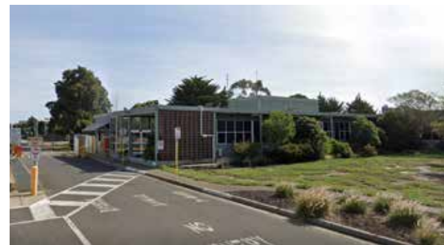
Image above: Entry to the existing site owned by Dow Chemicals, a designated SUZ3 area
